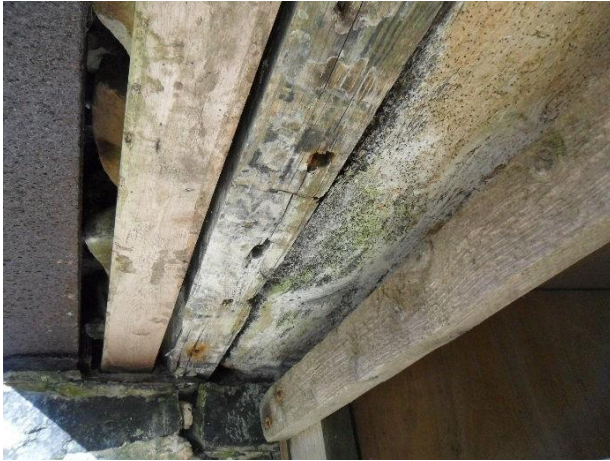
Inner lintels of south opening
