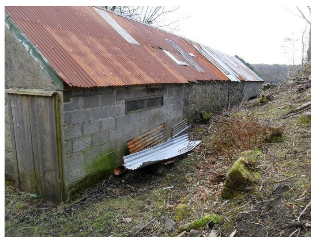
Rear view showing ground level; roof corrosion
