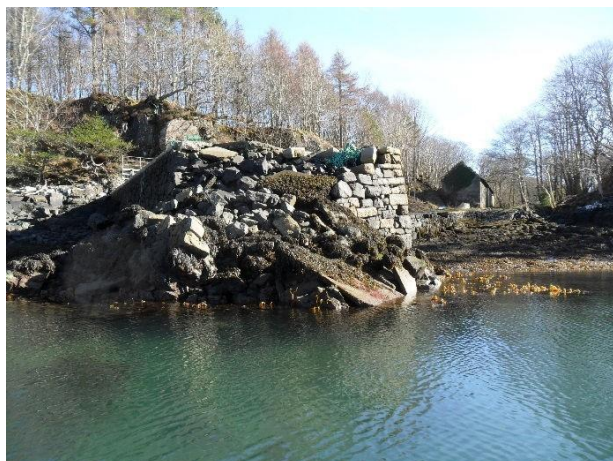
End of pier showing collapse
