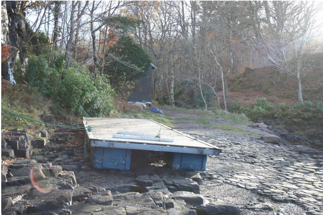
A section of pontoon owned by Tobermory Harbour Association is being stored on the slip. The slip is constructed of large, uneven, slippery boulders and filled with gravel.
