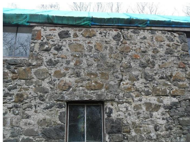
Cracking to west wall near windows
