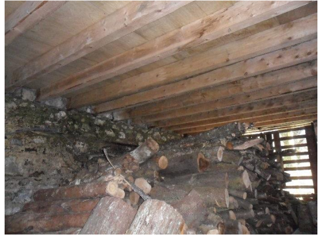
Floor joists at south end
