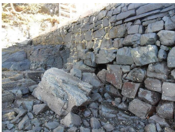
Pier north face at root showing pointing
