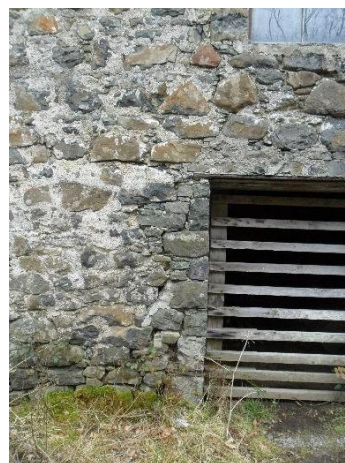
Vertical cracks adjacent to openings
