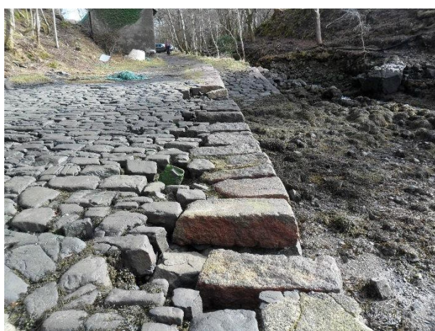
Displaced coping stones to wall
