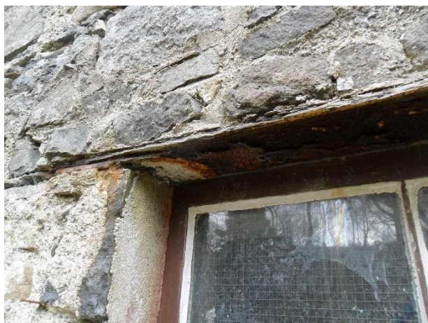
Corrosion to lintel; cracking to wall
