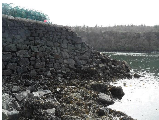
End of pier north face showing collapse
