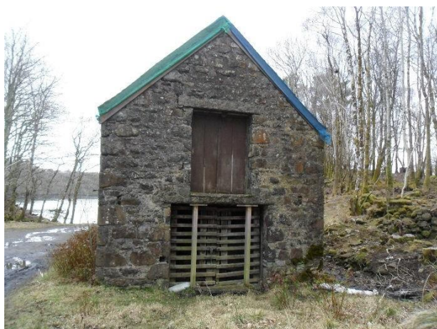
South gable: propped lintel; cracking upper lintel
