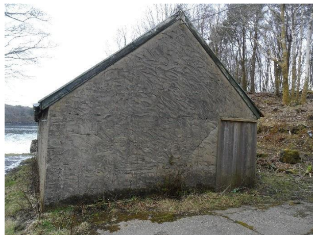
South gable showing crack at door
